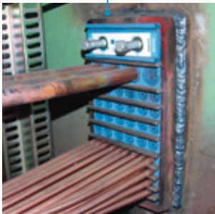
Roxtec S 6x1 for pressure-proof passage of copper pneumatic pipes in bulkheads onboard an FPSO.
