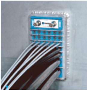
Roxtec S 6x1 frame transit for fire-proof sealing of cables through bulkhead onboard an FPSO.
