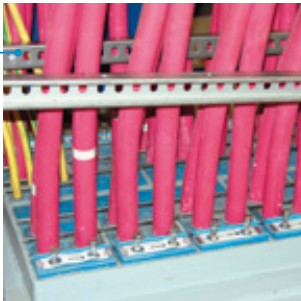
Roxtec SK 6+6x5 transit fire-proofing installation of power cables to the columns in drilling rig.
