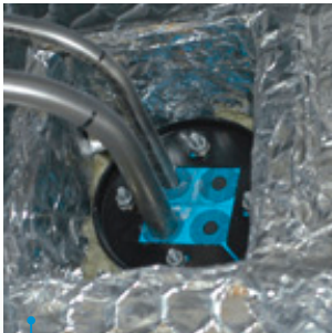
Roxtec R transit for passage and vibration dampening of several pneumatic pipes to door systems on drilling rig.
